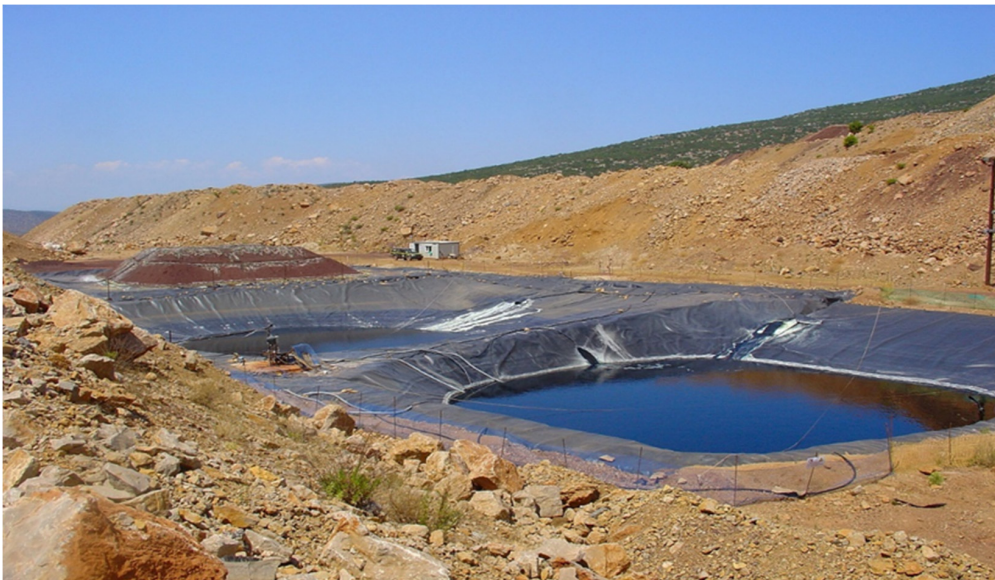
Scheme 1. General view of the heap leach pilot-plant.
